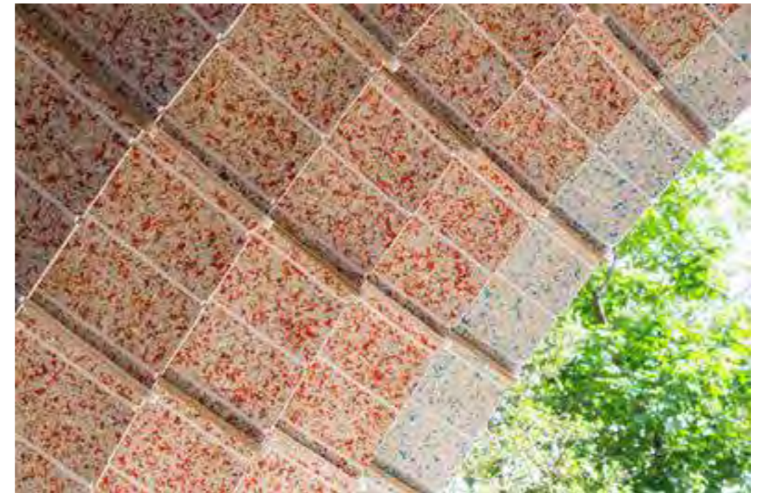
Fig. IV.5. 5. Reconfigured tetrapack material in the NO-WASTE-WALL NY, 2016, Hebel, Heisel, Block
