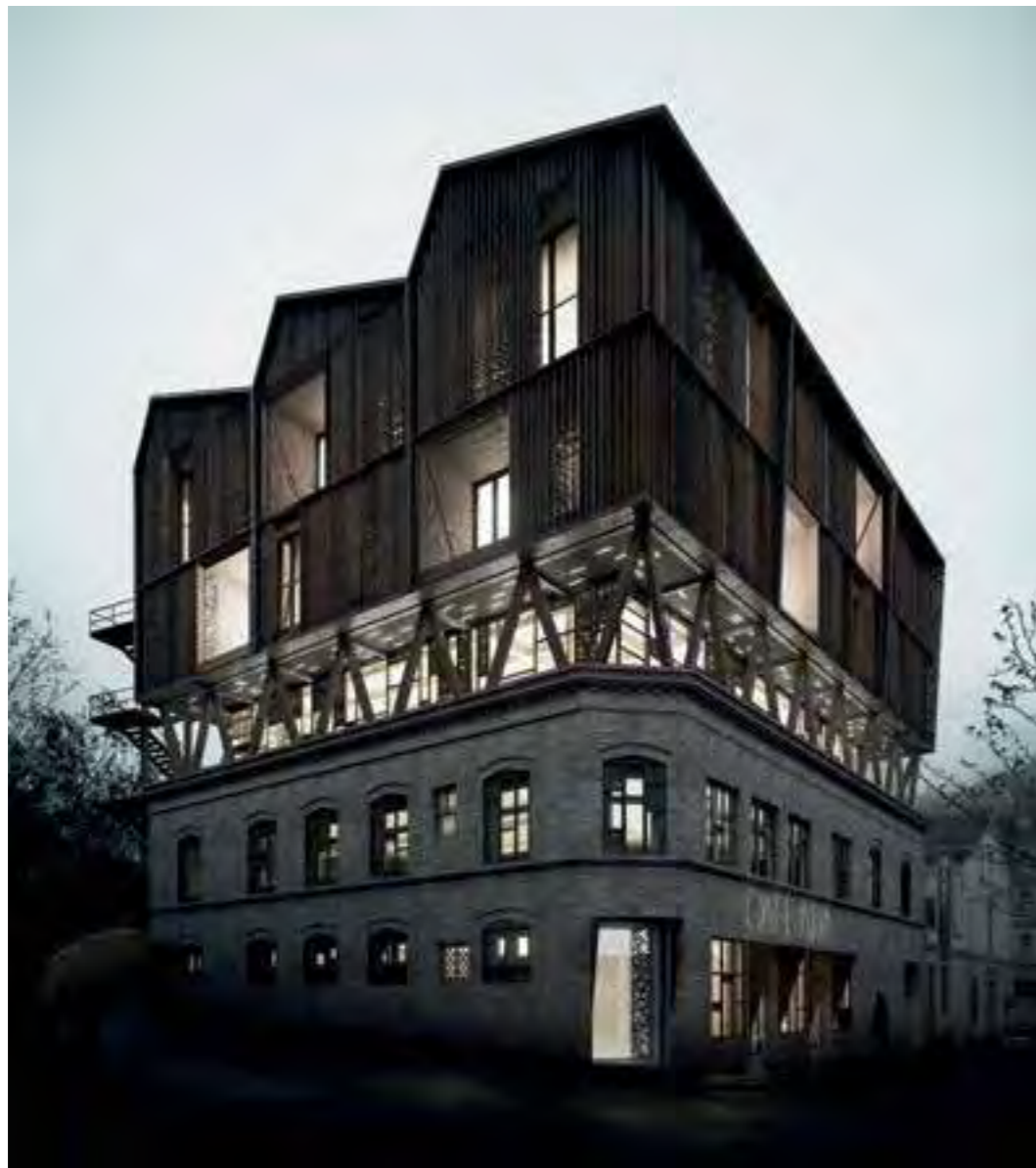
Fig. IV.1. 13. The overall design of RoofKIT as a top-up strategy for Café Ada
